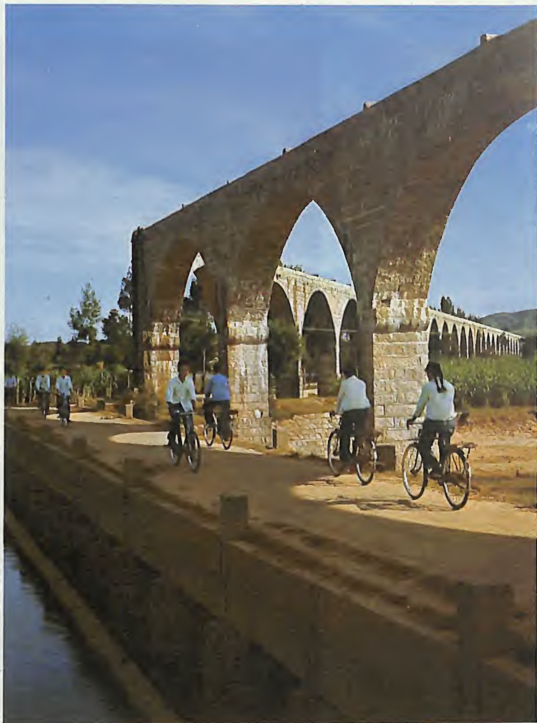
This 800-metre aqueduct was built by the joint efforts of two brigades.
